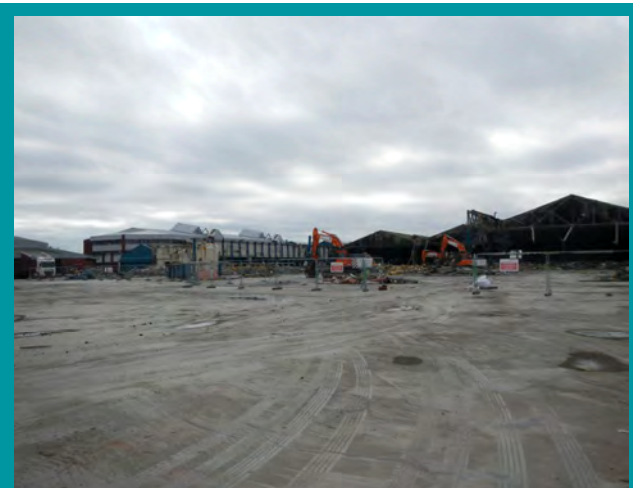
The Main Hangar under demolition.
