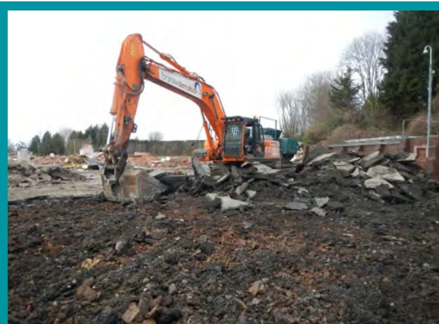
Hard-standing under removal.
